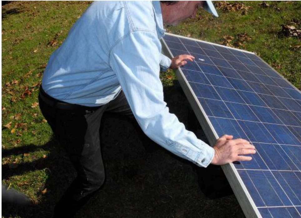
Figure 15. Worker pushing panel down into slots.
